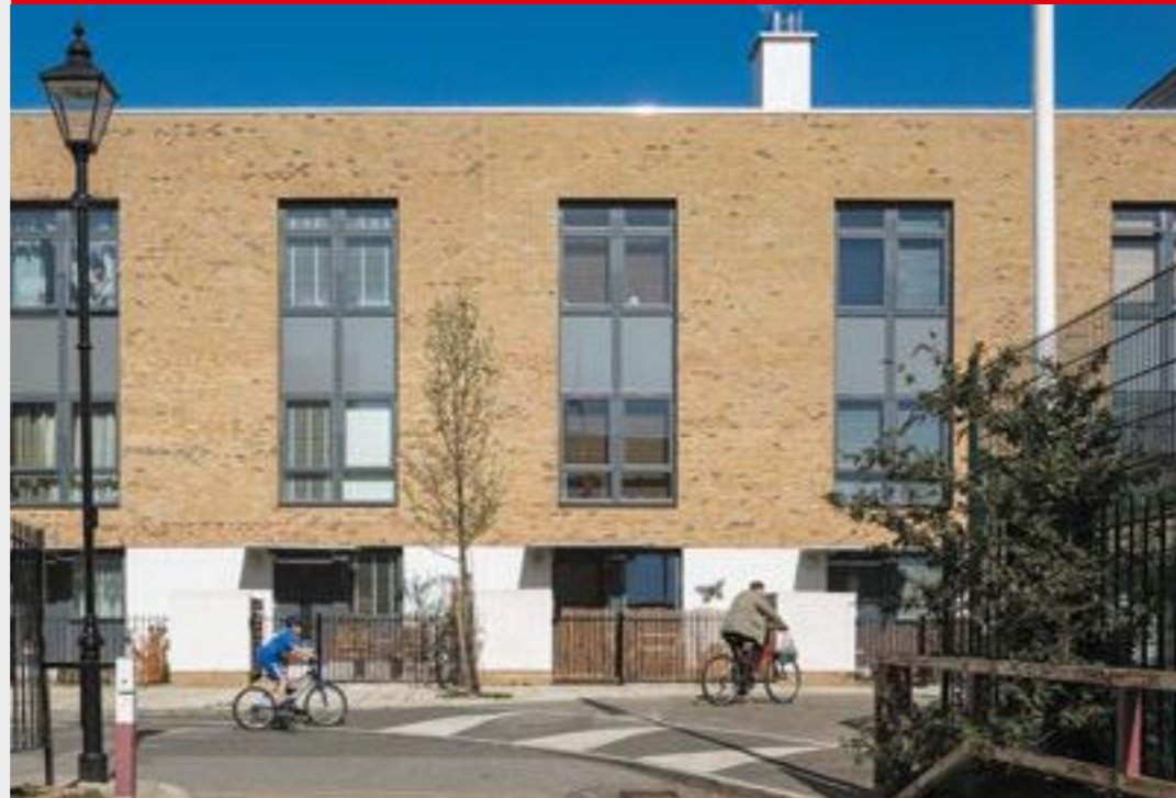
Photograph: Tim Crocker. Architect: Pollard Thomas Edwards
